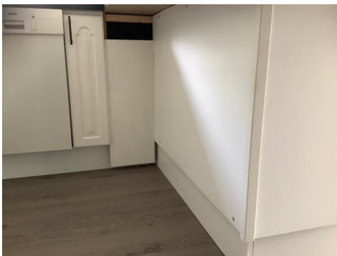
Foring/dekkside falt ned
