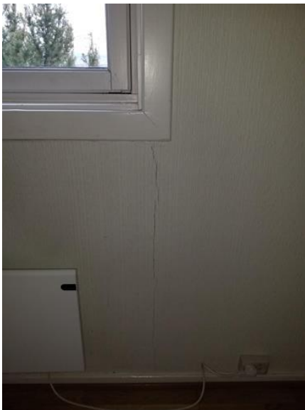
Overflater vegg - [Riss vegg stue. ]
