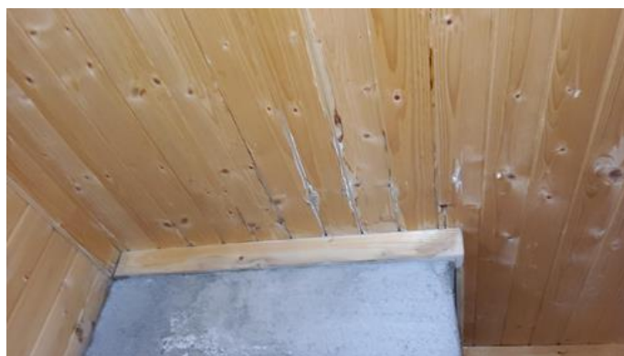
Overflater vegger / himling - [Gammelseterlia - Badstue - Himling (14.03.2024)]
