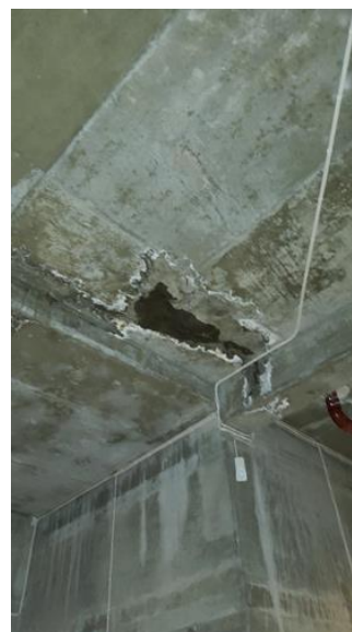
Overflater himling - [Gammelseterlia - U2 - Himling (14.03.2024)]
