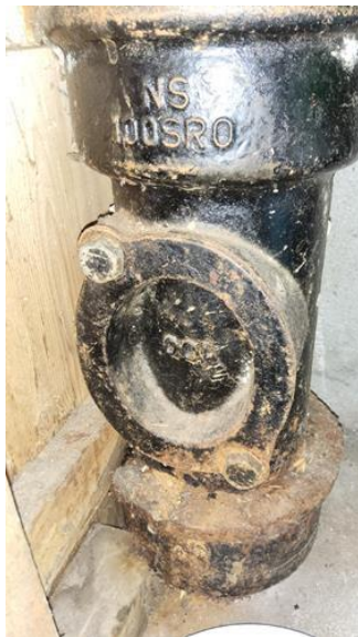
Stakeluke - [Stakeluke i kott under trapp ]
